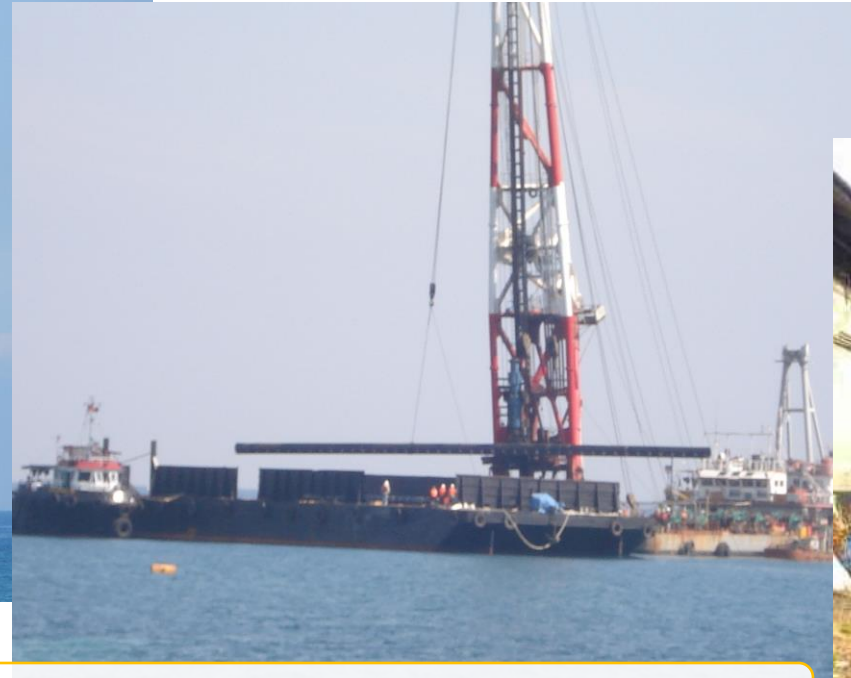
OFFSHORE PILING RIQ
